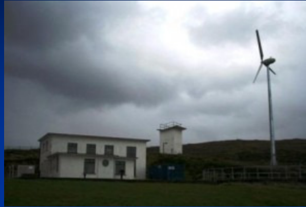
Energy audit on water treatment plant in Galway
