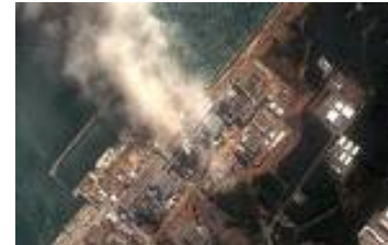
Smoke billows out of Fukushima reactor number 3 after Japanese earthquake and tsunami devastates the plant
